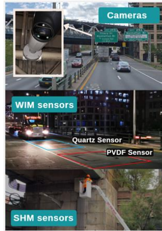
C2SMART Brooklyn-Queens Expressway Testbed
